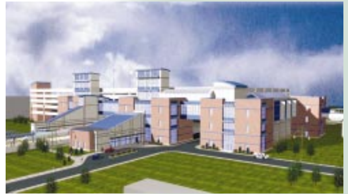
Warwick Intermodal Facility, Rhode Island Airport Corporation.
