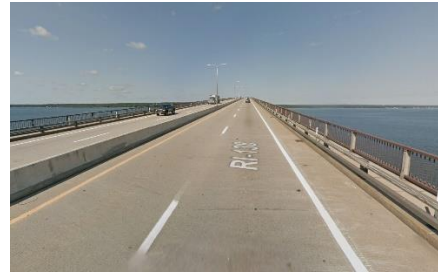
The Jamestown Verrazzano Bridge is legally open to bicyclists but is a significant barrier between Jamestown and North Kingstown
