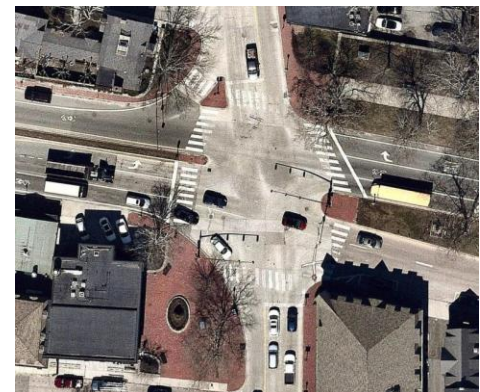
Large curb radii, vehicle slip lanes and discontinuous bicycle lanes at the intersection of Memorial Blvd and Bellevue Avenue creates a challenging intersection for bicyclists in Newport
