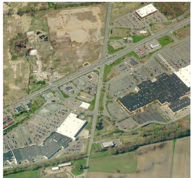
Lot-by-lot on-site parking requirements have created unnecessarily large parking areas in many areas, typified by the suburban shopping center.
