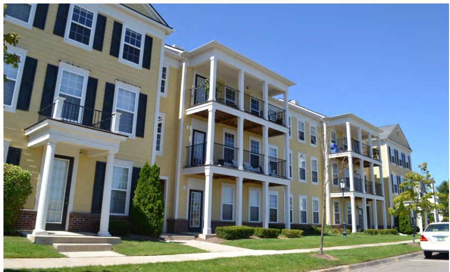
Diverse multi-family housing includes a range of offerings, from brick townhouses to three-story wood frame apartment blocks.
