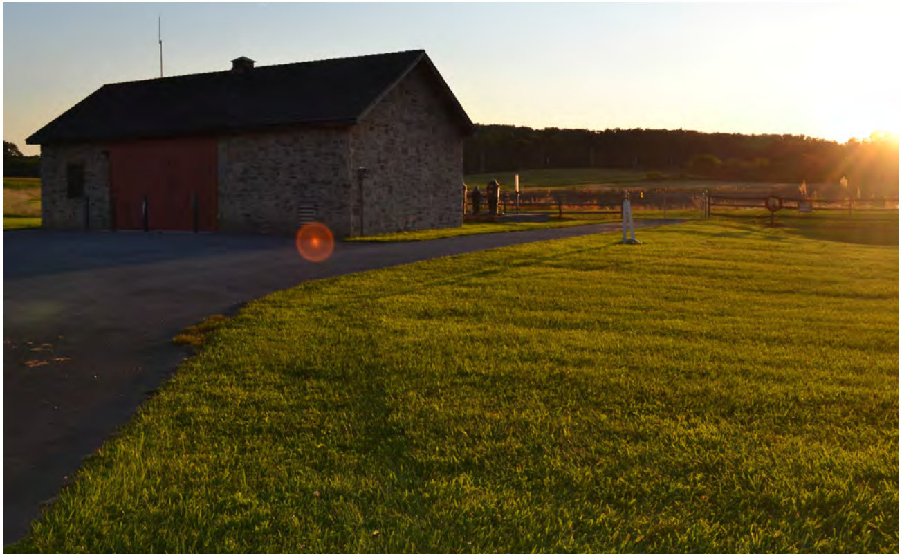
The agricultural landscape surrounding the project was largely preserved. Some of the hayfields are used to treat wastewater through spray irrigation.
