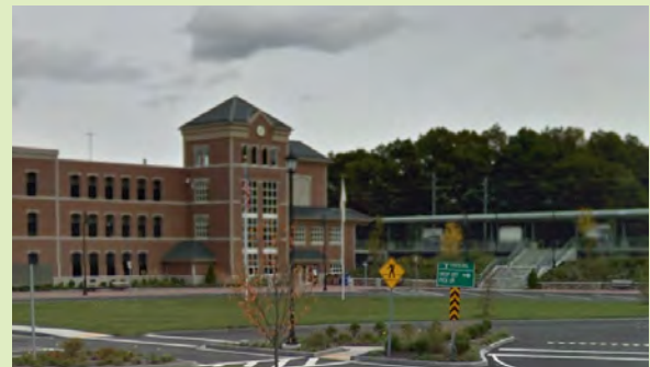
A new commuter station and parking garage is expected to drive demand for Transit-Oriented Development at Wickford Junction (photo courtesy Google Street View).
