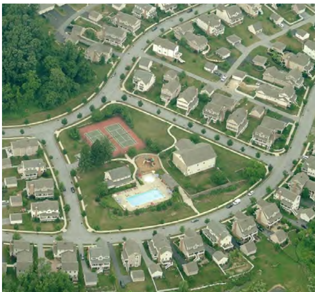
An historic farmstead and barn (above and right) were incorporated into the project as a community center complex with pool, playground, tennis courts and gardens (Aerial Photo Courtesy Bing Maps).
