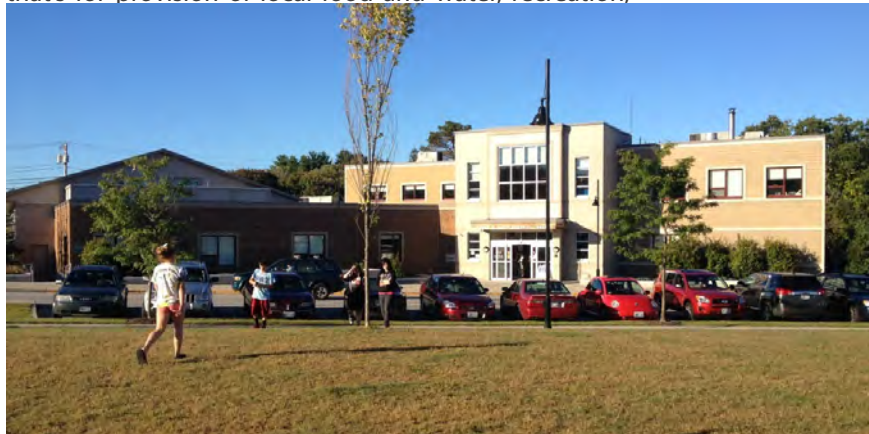
Redevelopment of the Stillwater Mill in Harrisville included a new community library (above), farmers market, riverwalk and community park. Amenities like these make the project more successful in the marketplace, but just as importantly, they enhance the quality of life for existing residents of the village.
