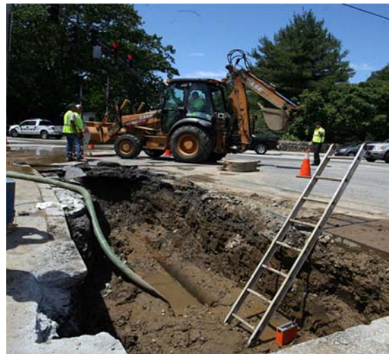
Fixing Water Main Leak, Westerly
