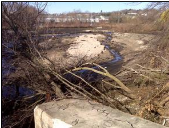
Geneva Pond after the dam ruptured in March of 2010.
