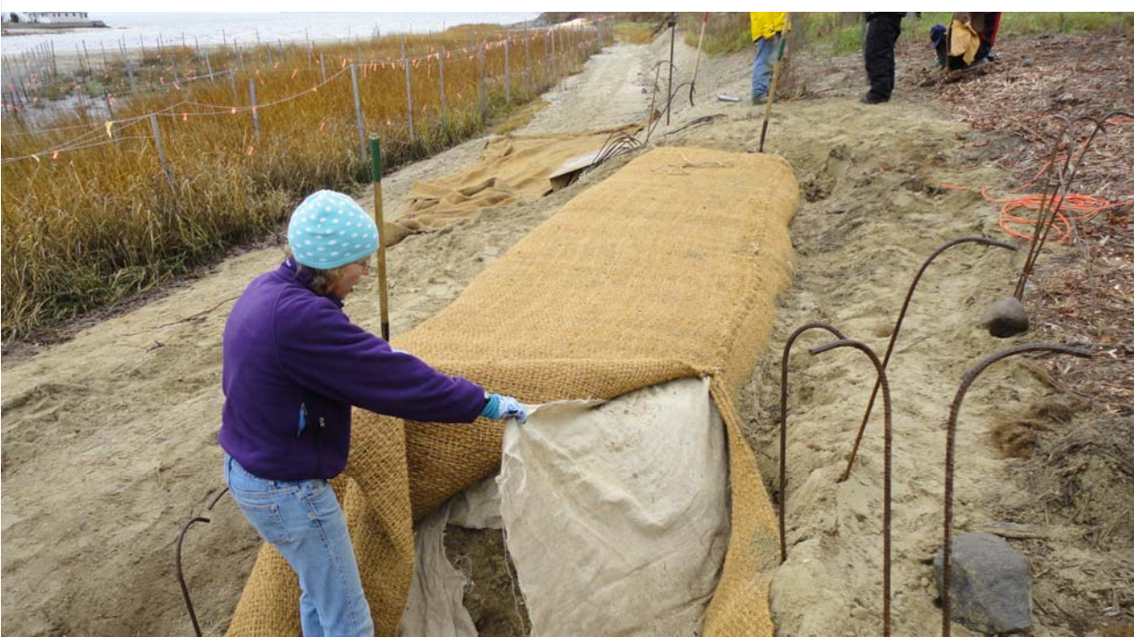
Figure 1. Shoreline protection project—Byway Road
