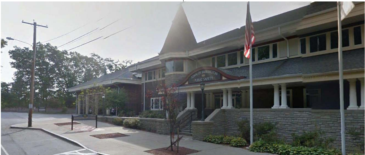
Public Safety Building, 100 Federal Road
