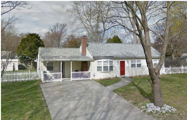
Figure 2: House Demolitions (examples)
