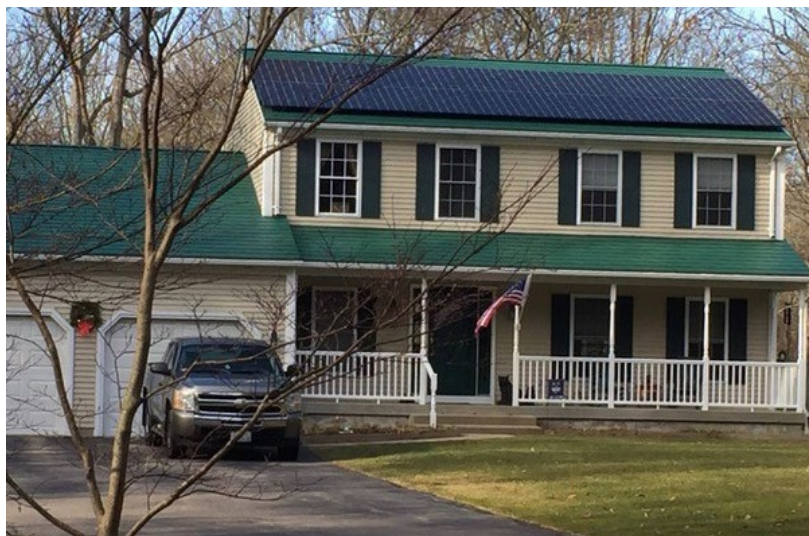
Frances Topping Charlestown Home with Rooftop Solar Panels
