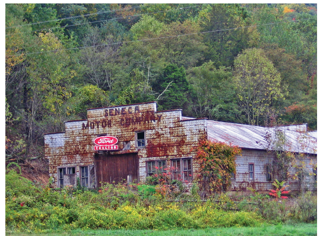
Photo courtesy of US EPA
