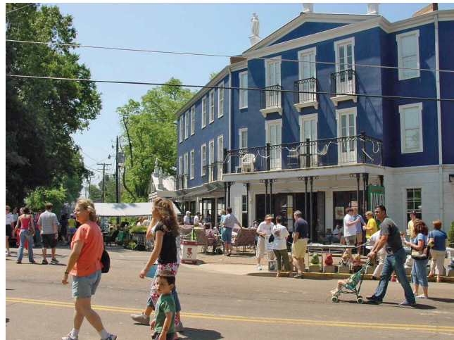
Photo courtesy of US EPA
