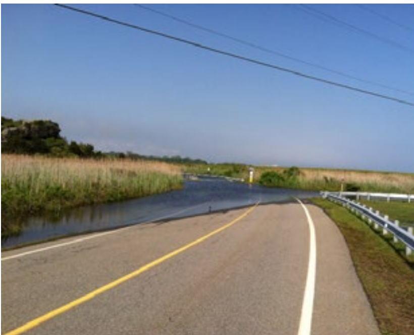
Figure 2: Flooding near Sauchest Point: June 2013
