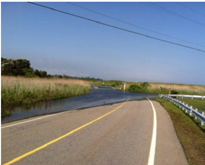
Figure 2: Flooding near Sauchest Point: June 2013
