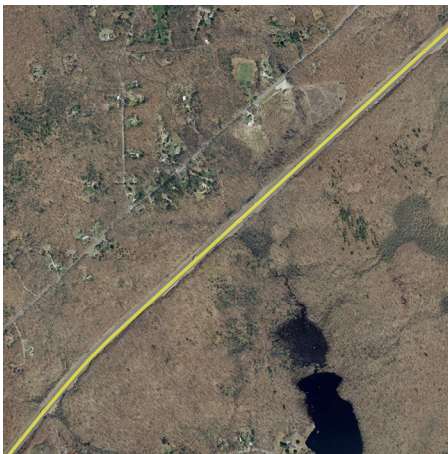
Roadway mobility: Interstate 95 in southern Rhode Island
