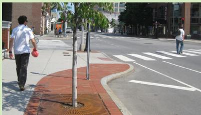
Curb extensions reduce turn radii and reduce turning speed.
