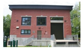
The Jamestown Public Water Supply system has a pre-treatment facility at South Pond. This facility was designed to provide chemical treatment for disinfection, taste, and odor control, color reduction, pH adjustment, and flow monitoring. This facility has the capability to treat up to 500,000 gallons per day with the existing chemical feed pumps amestown Water Treatment Facility
