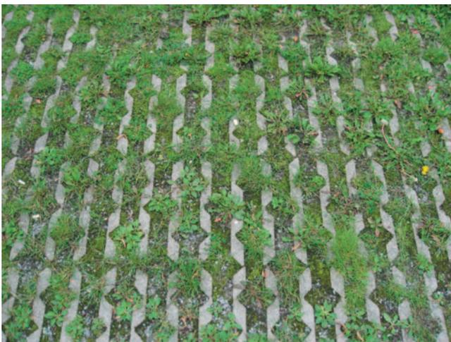
New kinds of porous or pervious pavers can allow water to infiltrate into the soil while still supporting heavy use
