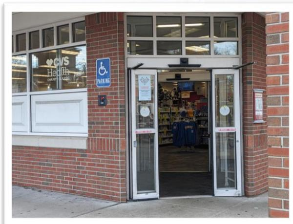
**Figure 13: The front doors of the CVS in the Barrington Shopping Center, serving as an example of a vulnerable entry point where floodwater may infiltrate a critical building during a flooding event**
