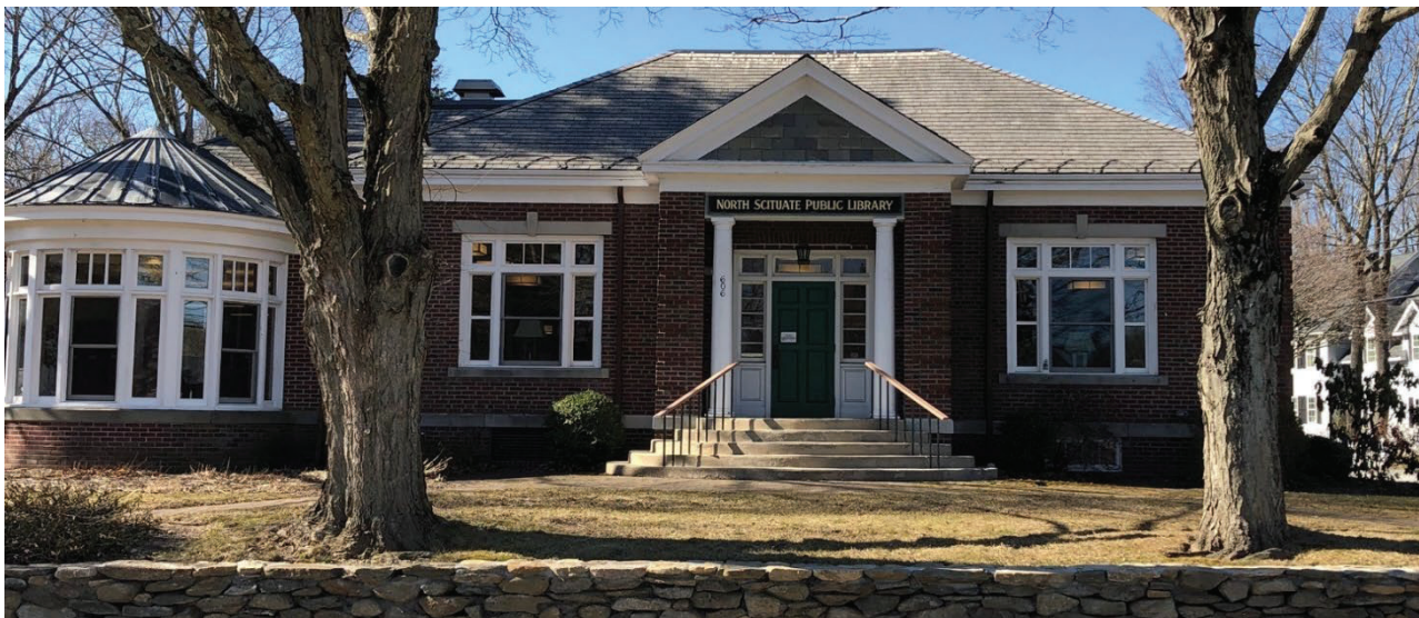
Figure 10-2. North Scituate Public Library
