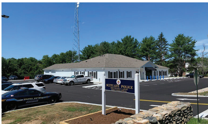
Figure 10-1. Scituate Police Station (Sugrue & Associates, Inc.)
