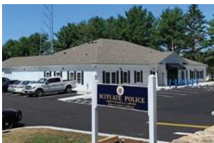
Figure 1. Scituate Police Station (Sugrue & Associates, Inc.)
