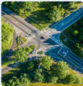
Vegetation near Intersection
