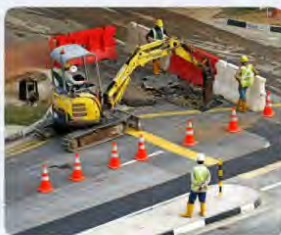
Intersection Realignment Photo courtesy of Ceogh/Freerange Stock
