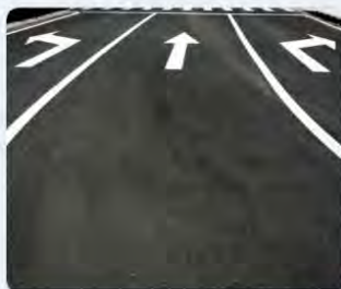
Dedicated Left and Right Turn at Intersections
