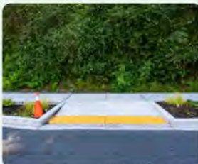
Curb Ramps/Sidewalk Utility Coordination
