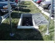
LID using vegetation and structures to mimic pre-existing hydrologic conditions
