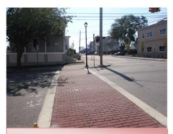
Stamped asphalt is less expensive than concrete and is attractive
