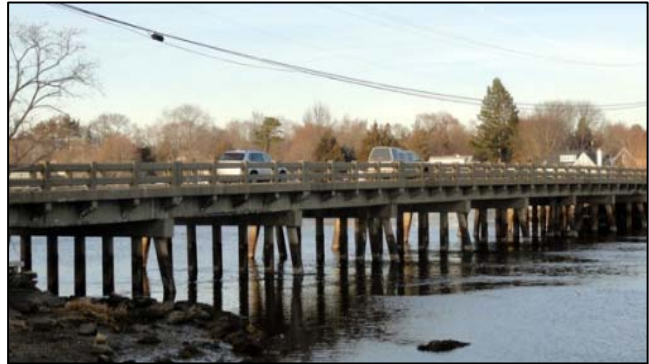
Central Bridge 182 in Barrington will be rebuilt with sea level rise in mind.
