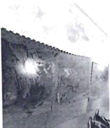
Charlito Middle School has signs of water ingress at several locations throughout the building. Exploratory analysis/repair is needed.
