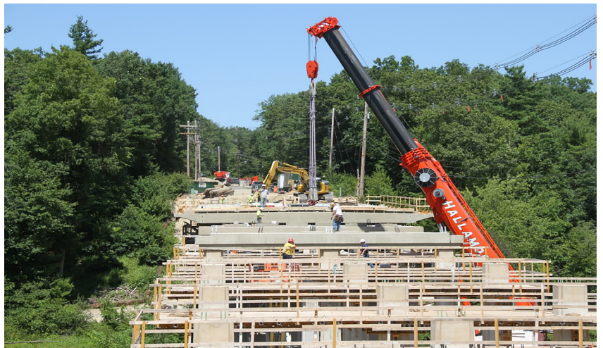
Image 12: Replacement of the Stillwater Viaduct
