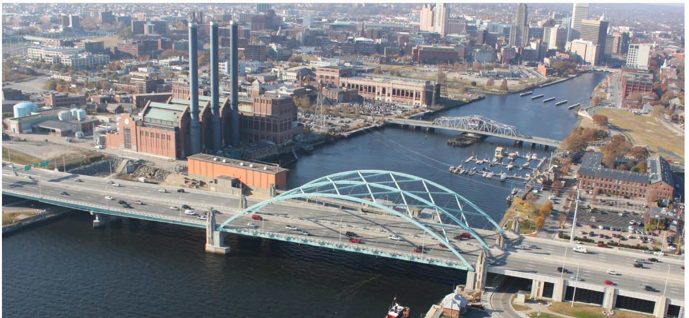
Image 11: View of the IWay in Providence
