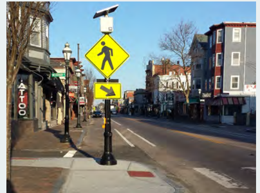
Pedestrian signs were installed making crosswalks more visible
