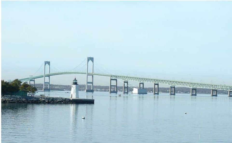
Pell Bridge, Newport
