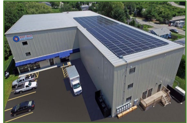
77.3 kW Solar Energy System, Storage Facility, Middletown, RI
