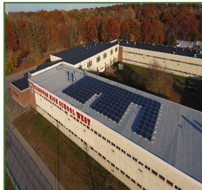
51.3 kW Rooftop Solar Energy System, Cranston High School. Cranston, RI
