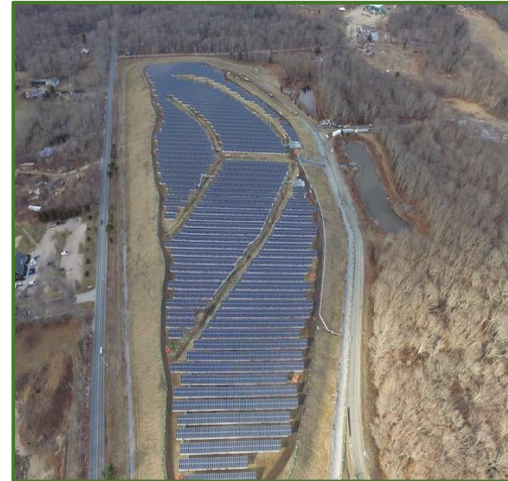
4.7 MW Solar Energy System, Rose Hill Closed Landfill, South Kingstown, RI
