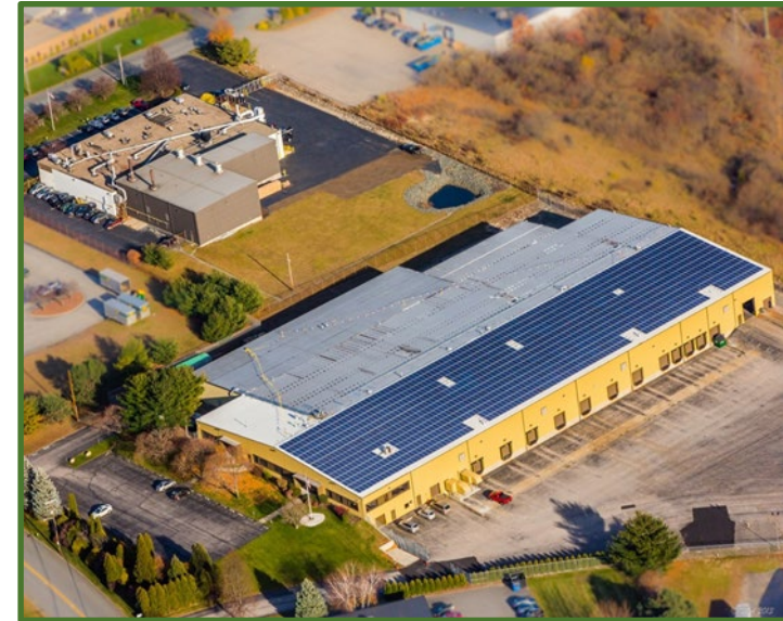
500 kW Rooftop Solar energy System, Gannon and Scott Recycling, Cranston, RI
