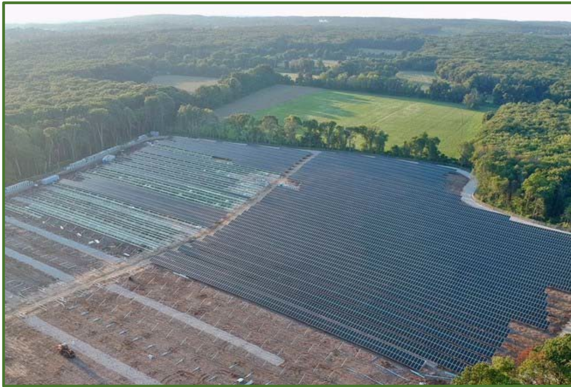
Southern Sky Renewable Energy, 21.3 MW, Gold Meadow Farms, Cranston, RI (Conti Solar)
