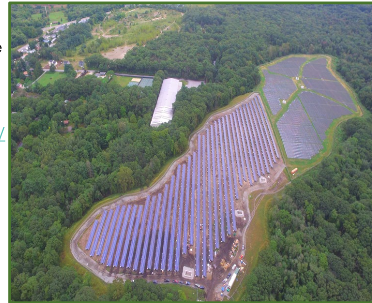
7.71 MW Solar Energy System, Closed Landfill, East Providence, RI
