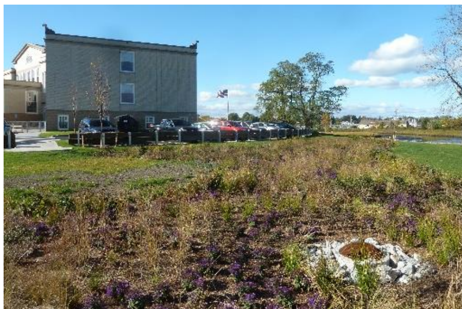
Bioretention areas at Guiteras School
