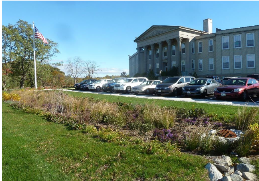
Completed bioretention project at Guiteras Elementary School
