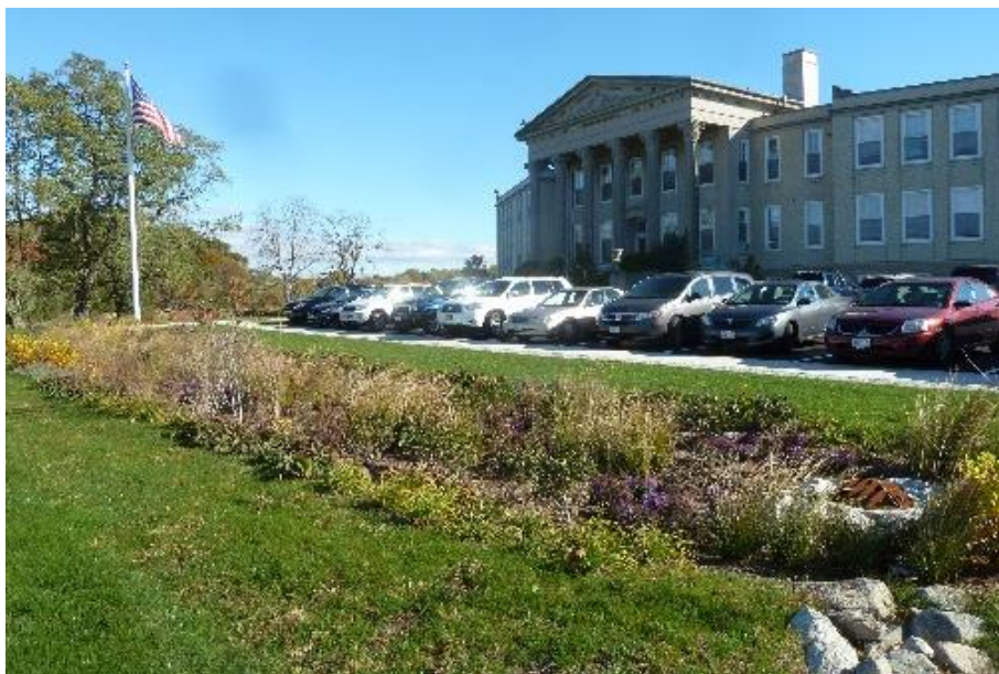
Bioretention areas at Guiteras School
