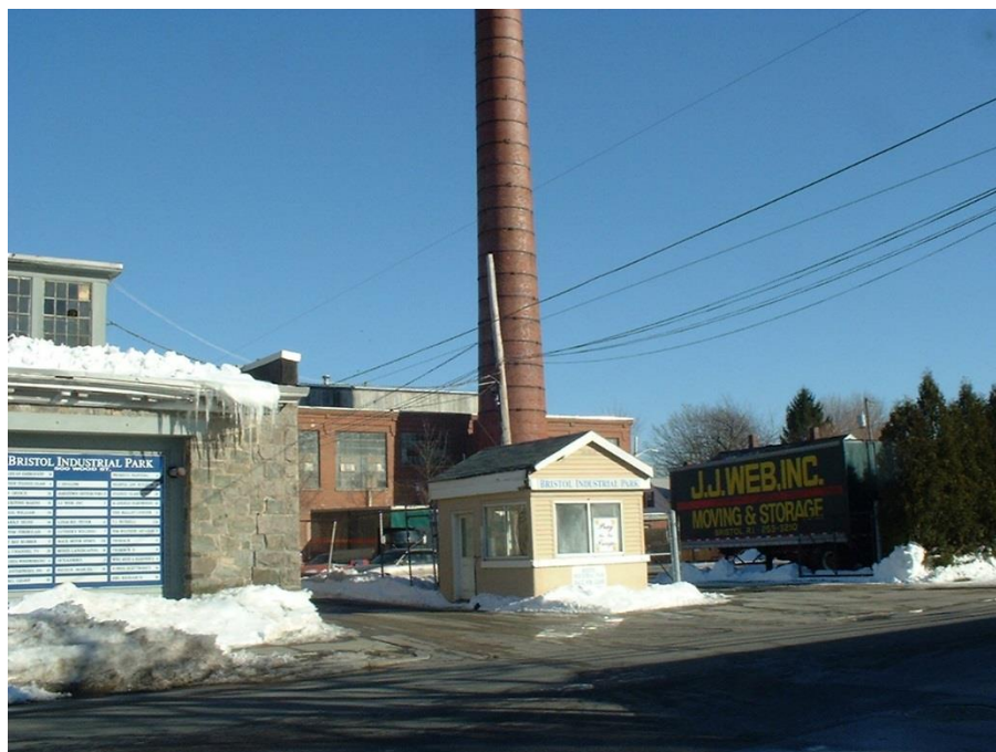
Bristol Industrial Park
