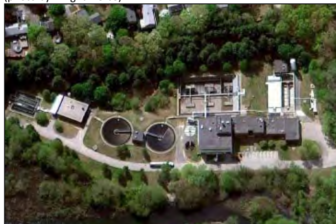
Figure SF-14: Smithfield Water Pollution Control Facility (photo by Wright Pierce)
