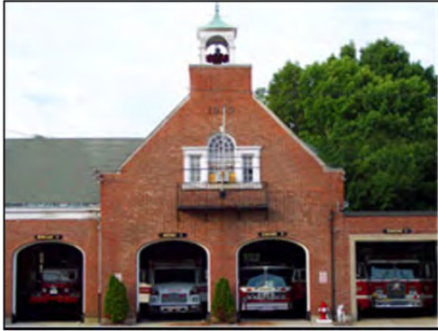
Figure SF-4: Fire Department Headquarters
