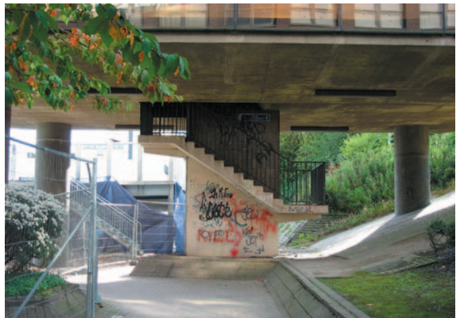
This underpass in Cumbernauld, Scotland, is cut off from natural surveillance
