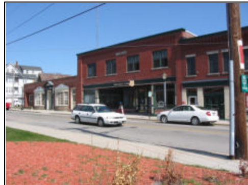
Renovations are underway at this Railroad Avenue building located across from the Westerly Station.
