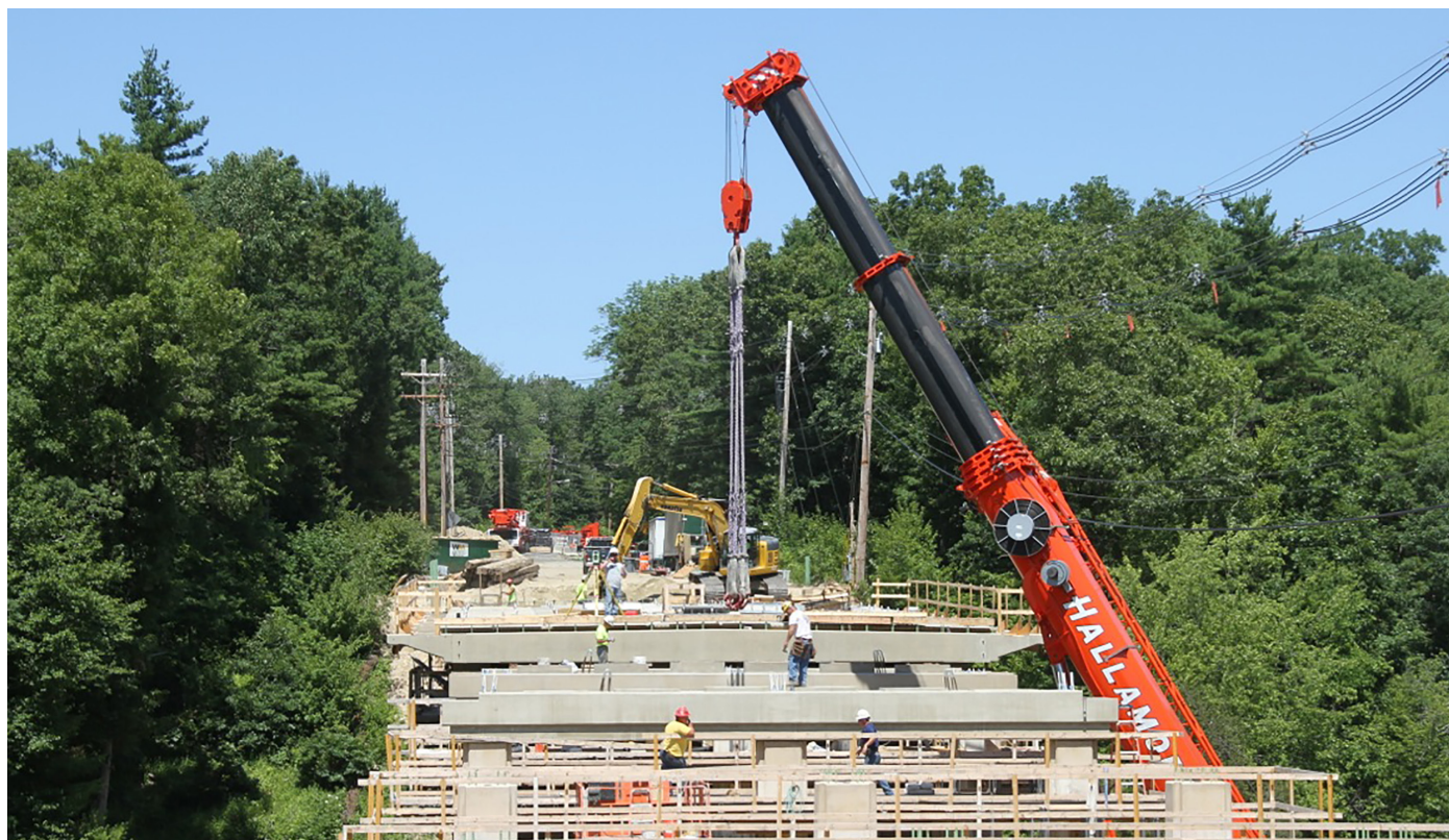
Image 12: Replacement of the Stillwater Viaduct
