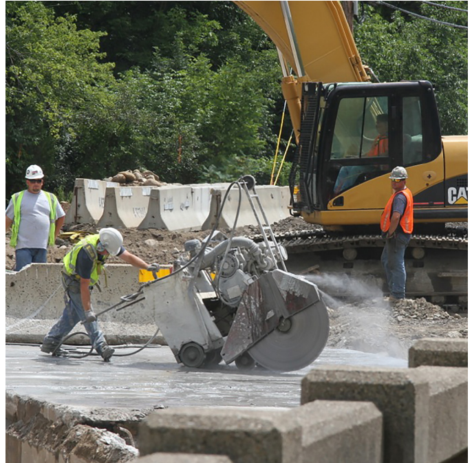
Image 1: Frenchtown Brook Bridge
