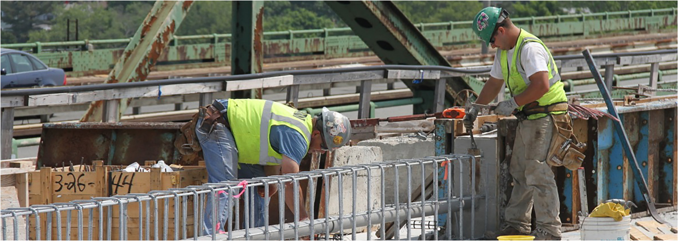
Image 2: Sakonnet River Bridge Construction
