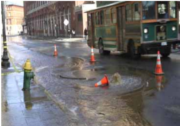
Water Main Leak, Sabin Street, Providence 2010
