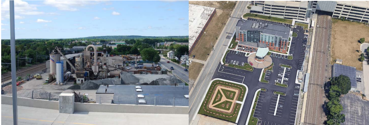
Hyatt Place Hotel: Before /After
